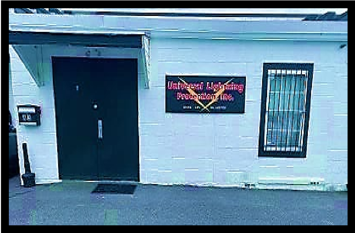
FRONT OF BUILDING
