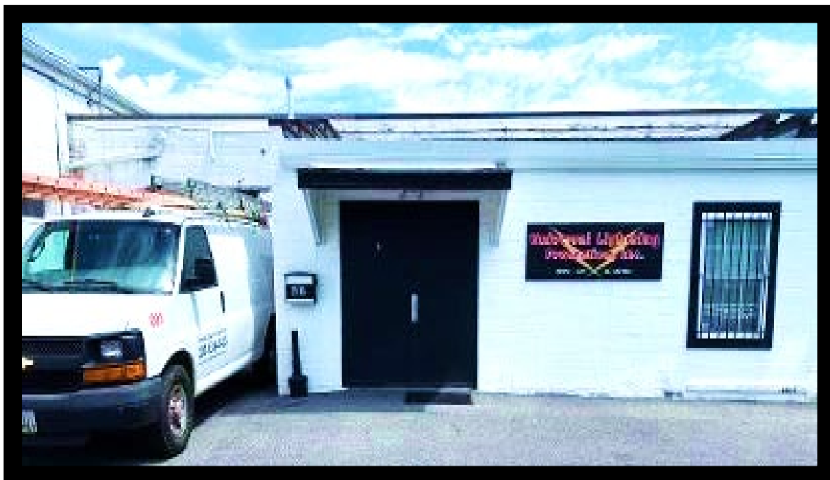
FRONT OF BUILDING
